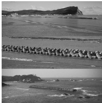
Fig. 1 - Concrete modules deployed as shallow water artificial reefs and wavebreakers. All photos H.K. Marshall.
